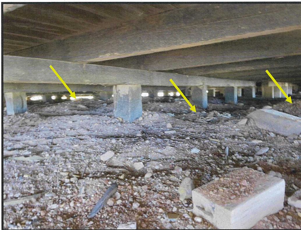
Photograph 17 – Variation of ground surface levels in the subfloor space.
