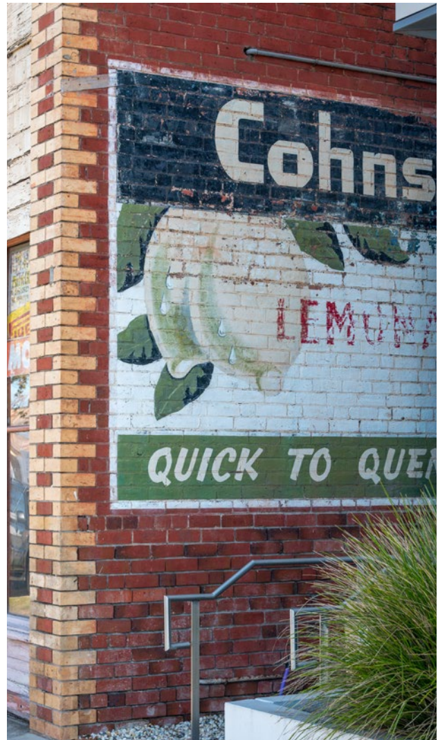
Figure 29: Example of signage located on side walls.
