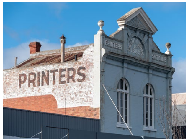
Figure 33: Victorian-era building with raised cement lettering in the parapet and a historic 'ghost sign' painted onto the side elevation.
