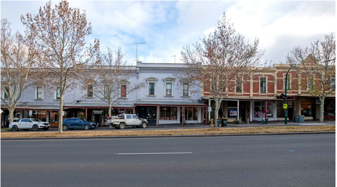
Figure 9: A row of shopfronts at View Street, Bendigo with simple reconstructed verandahs, stepped to follow the street grade. The simplified interpretation of Victorian-era verandahs and visual cohesiveness helps maintain the local character.
