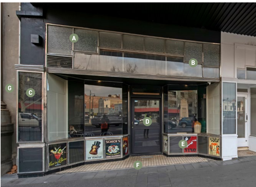
Figure 39: Typical Interwar and Wartime building.
