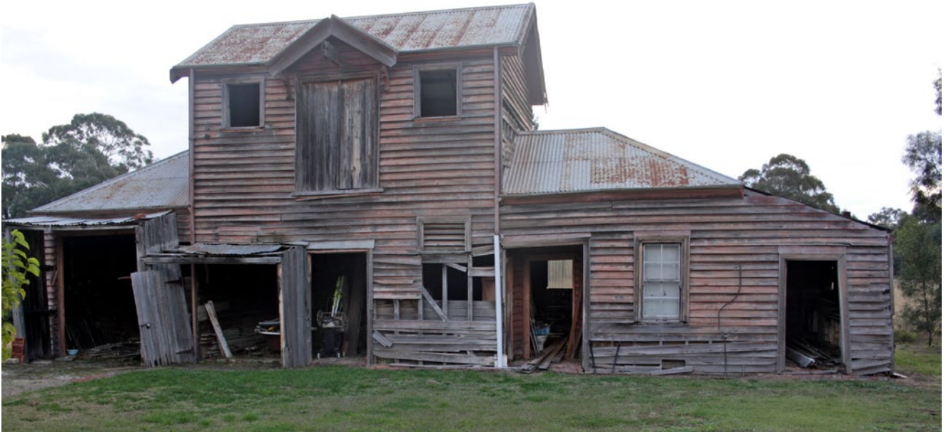
Figure 13: The Stables, prior to restoration works.
