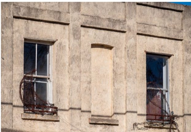
Figure 22: A building that has an unpainted render finish on the parapet, which contributes to its character and intended appearance.
