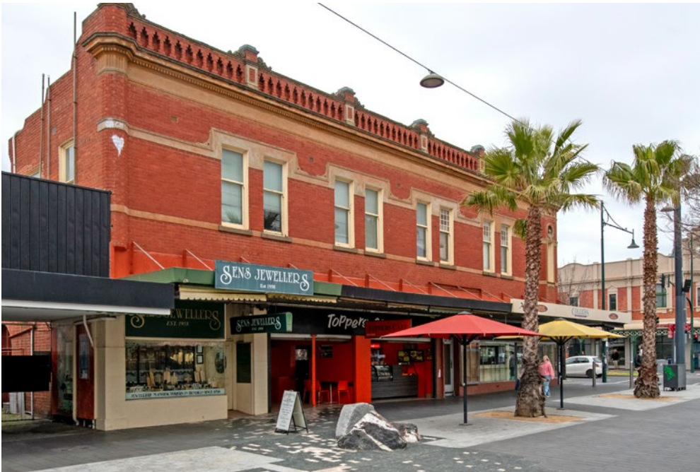
Figure 20: Signage is appropriately contained within the extent of the awning fascia board. Secondary signage has been placed inside the glazing on the toplights above the shopfronts.
