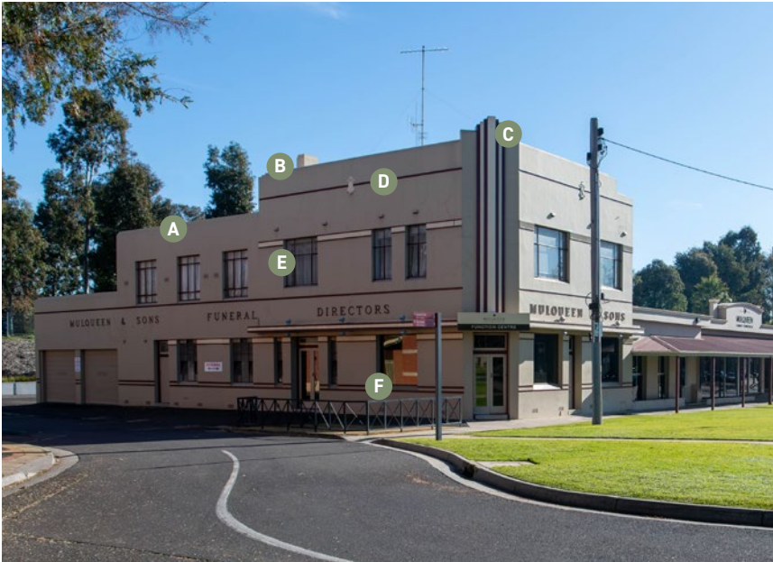
Figure 38: Typical Interwar and Wartime building.
