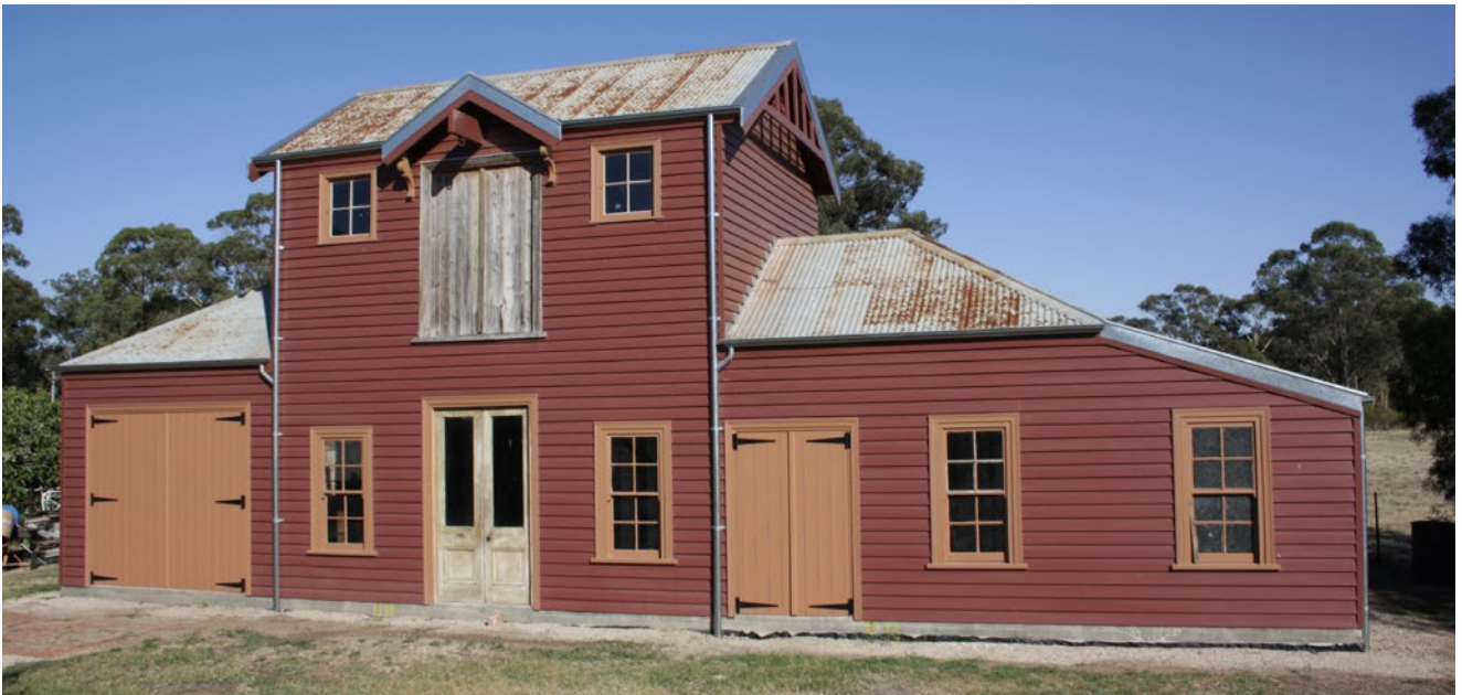
Figure 14: The Stables, following reconstruction .
