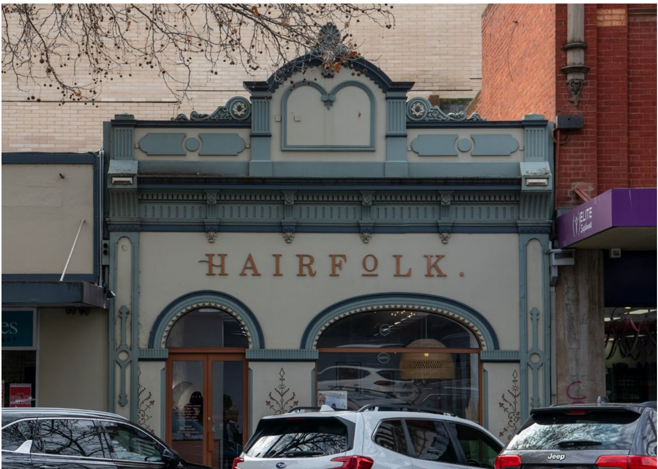
Figure 24: This Victorian-era shop has been painted in a compatible modern colour scheme. While the colours were not particularly common for exteriors during the Victorian period, they are generally muted shades within the light-to-mid tonal range. The updated colour scheme highlights the detailing in joinery and moulding, referencing Victorian-era trends. Despite not being historically accurate, the colours are considered sympathetic and appropriate.
