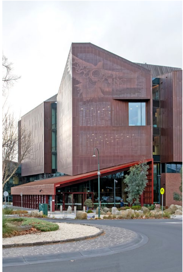
Figure 12: The Bendigo Law Courts demonstrates architectural quality through its striking contemporary design and consideration of local context. The design incorporates strategies to reduce its visual dominance, including balancing solid-to-void ratios, incorporating projecting and recessive elements, and a human-scale, sheltered podium at ground level.
