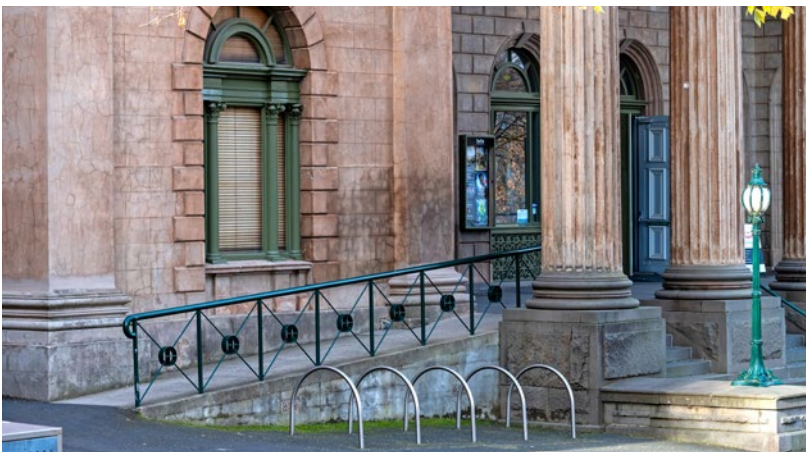
Figure 16: The Capital Theatre, Bendigo, features a sympathetically designed ramp that provides equal access to the primary entrance.
