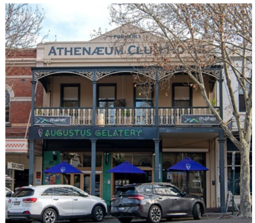
Figure 10: Restoration of former Athanaeum Club verandah. The historic black-and-white photo reveals the original design and was used to inform the reconstruction of the verandah.
