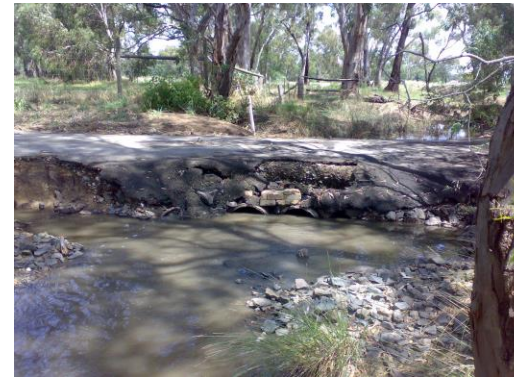
Viola Road Crossing location – 2011 Pre works
