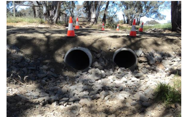
Viola Road Crossing location – 2017 Post works
