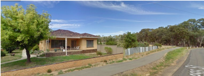
Furness St – West of Hammill Street
